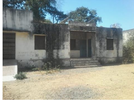
Health Sub-Centre, Pal
