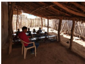
Anganwadi Centre operational in kaccha premises
